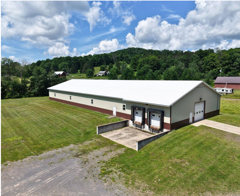
Existing Conditions at 5 Grant Pl
