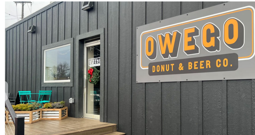
Local businesses that opened with support of DRI funding in Owego (2018 DRI)
